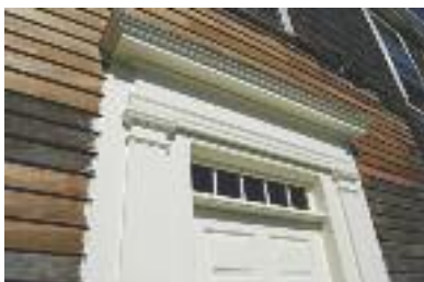
Entrance door and surround by Matthew Diana, PC '10
