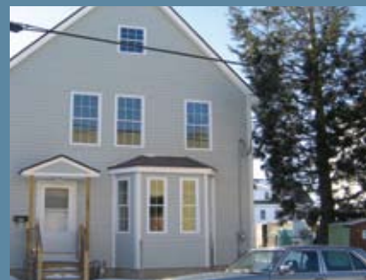
AFTER: With the help of NBSS volunteers, the homes were rebuilt and will be occupied this spring.
