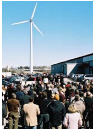
A 600KW WIND TURBINE is now providing power for Mark Richey Woodworking , Newburyport, MA, where Greg Profido (CF '88) is COO.
