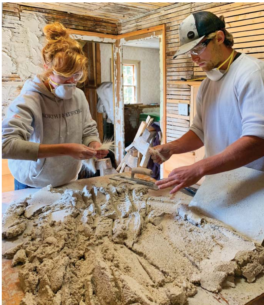
Two students in the 2019 Preservation Carpentry program mix horsehair plaster to apply to the lath walls behind them. Even before the pandemic, students often wore masks to work with some materials. Off-site projects like these are a core part of their curriculum.
