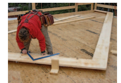
Transfer the stud layout
